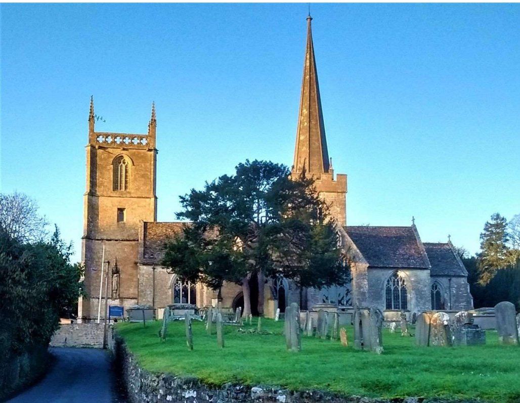
St Mary's Purton exterior view
